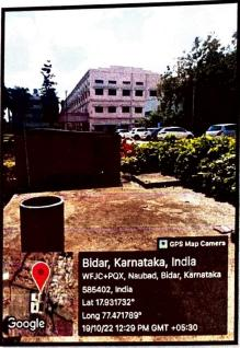
A water tank has been constructed in the college campus of capacity 30,000 litters of 10x10 sqft and also motor of 5 HP has been installed to pump the water
